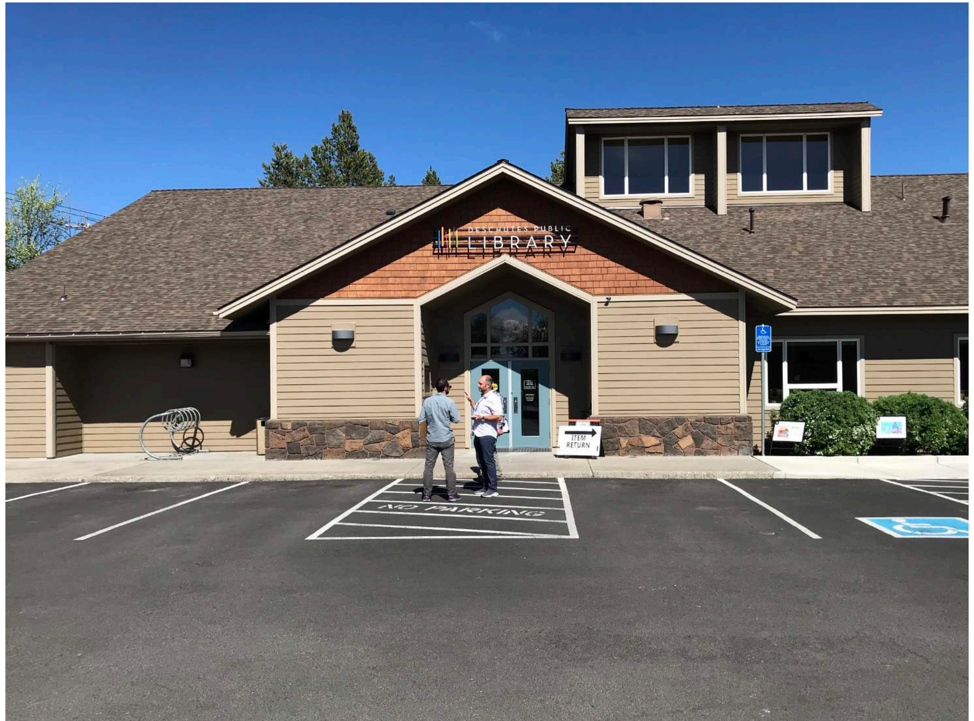
La Pine Library main entrance
