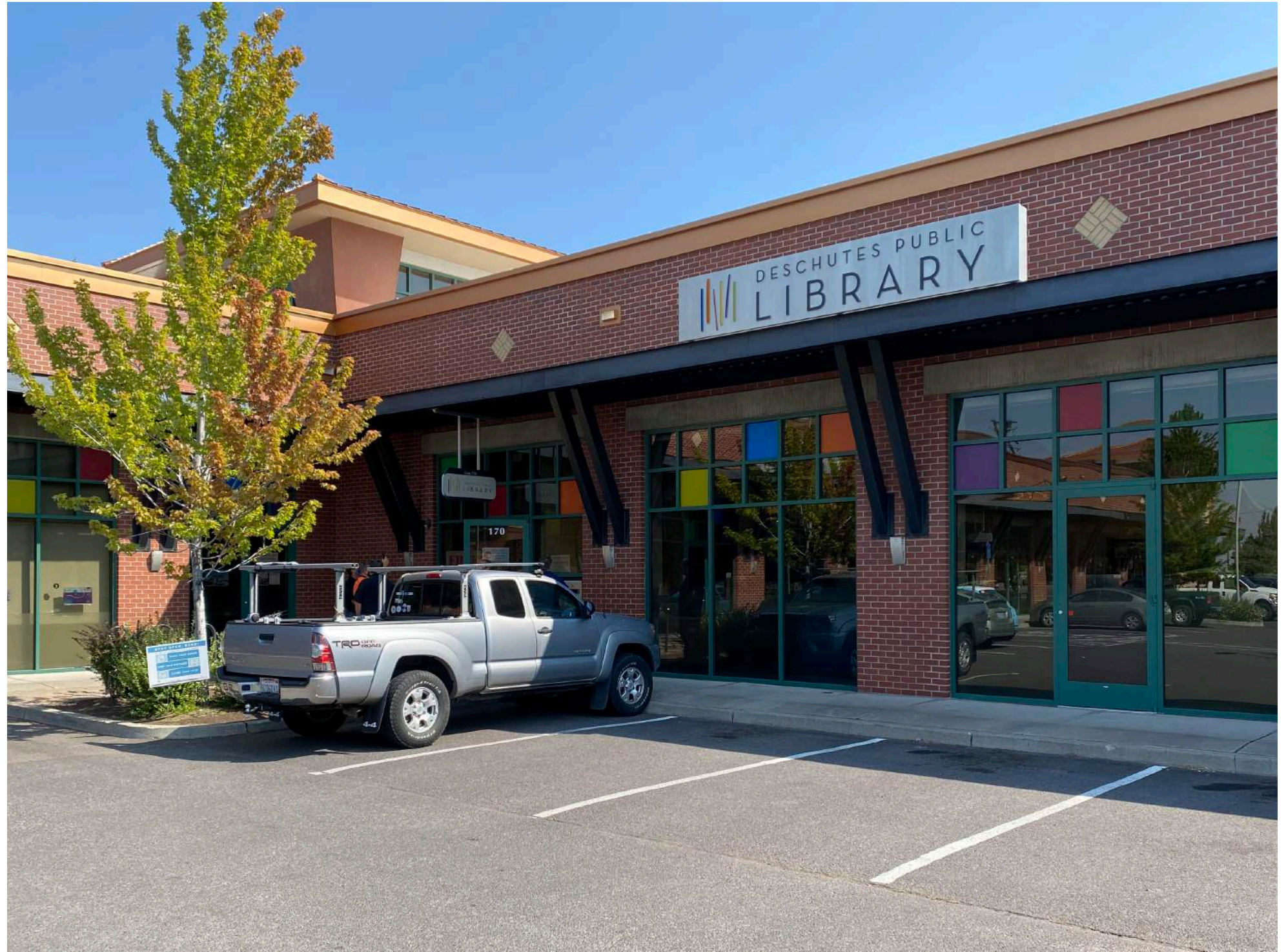
Library main entrance
