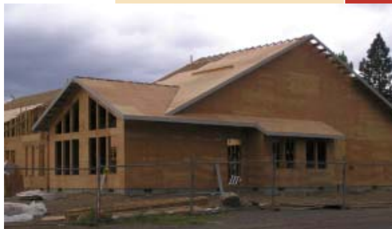
The new Sisters Public Library currently under construction.
